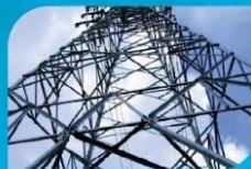
Latis Towers (Power & Telecommunication)
