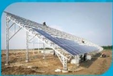
Solar Structures & Other Steel Fabrication Work
